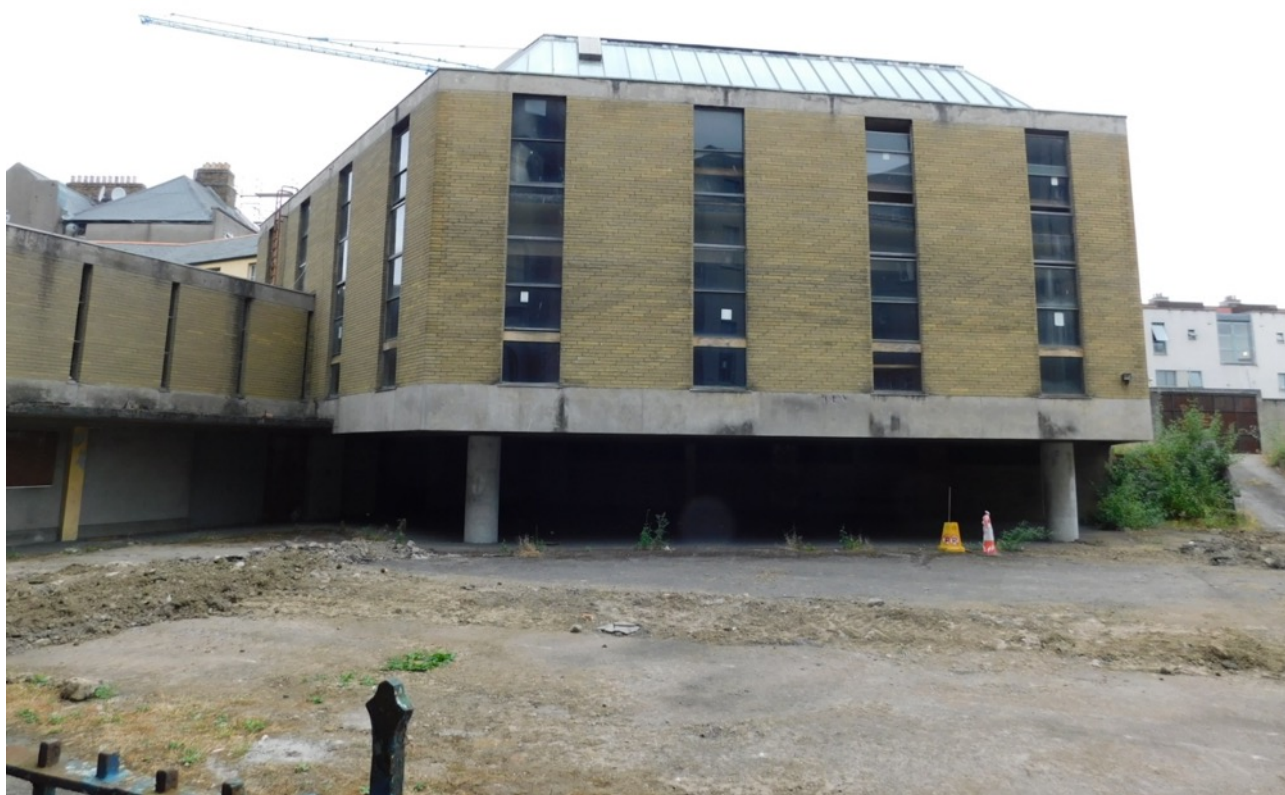
Figure 5.3.21: The Hexagonal Amharclann Building from the yard area.
